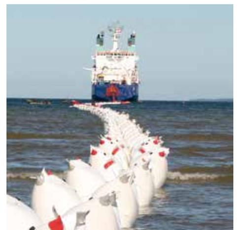
Image to the right: Laying the Estlink HVDC Light cable 2x75 km. The cable connects Estonia with Finland.
