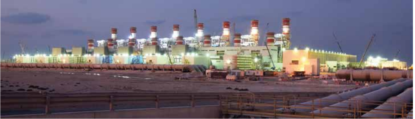
Image above: The Ras Laffan power plant and desalination works in Qatar. This is the largest installation of its kind in the country, with capacity to generate 2,730 megawatts (MW) of power, and produce more than 286,000 cubic meters of potable water per day.
